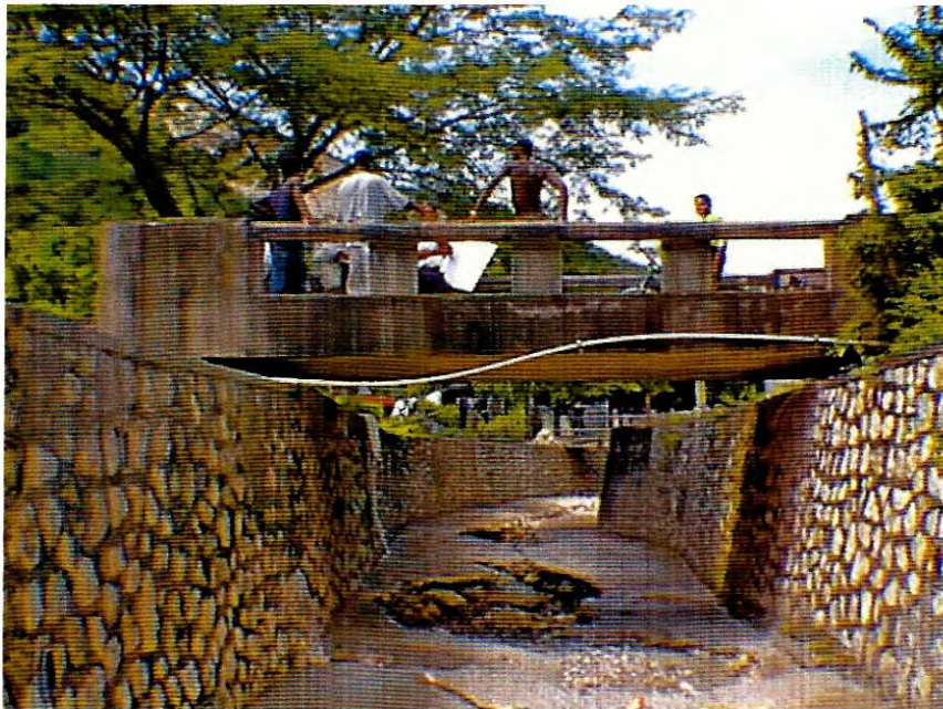
Plate 2. Bridge exposed to scouring of gully channel near confluence with Hope River.
