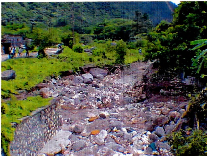
Plate 4. Downstream view of section of gully embankment that was damaged by flood water overflow.
