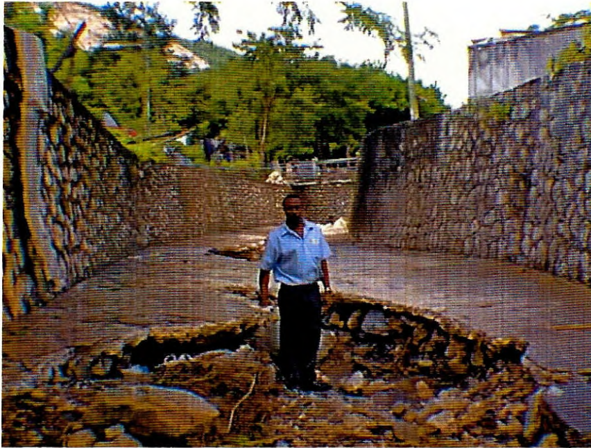
Plate 1. Scouring of concrete channel of Lower August Town Gully near confluence with Hope River (Section 1).
