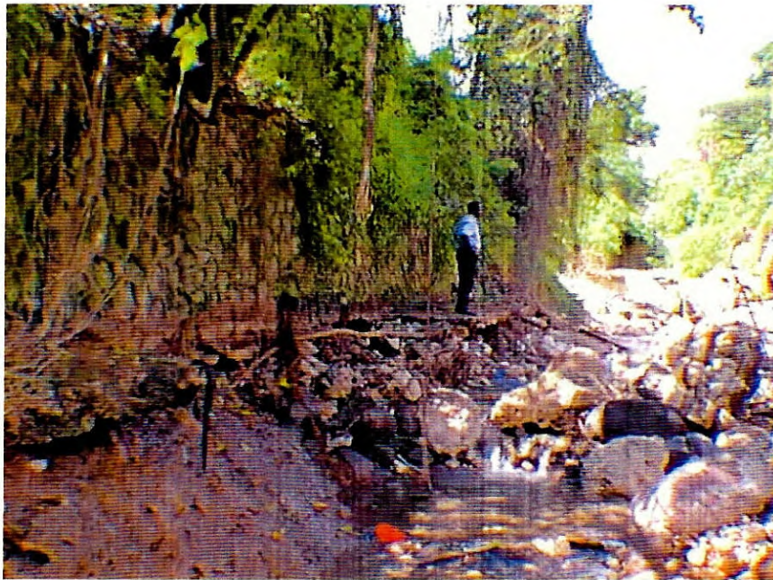
Plate 6. Undermined gully wall caused by erosion of the gully channel (Section 3).
