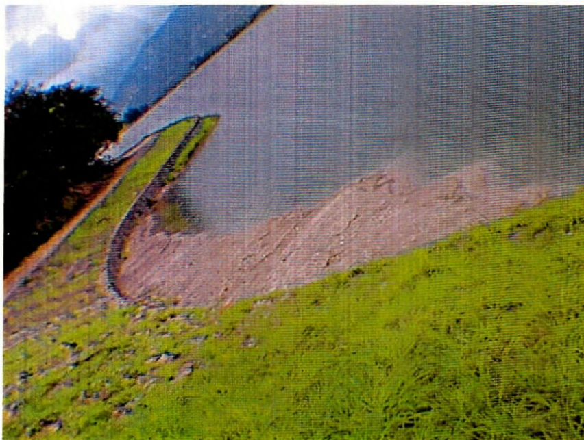
Plate 12. Quarried material deposited in the Mona Reservoir after heavy rainfall (6 November 1998).
