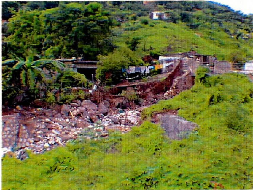
Plate 3. Upstream view of collapsed gully retaining wall (Section 2).
